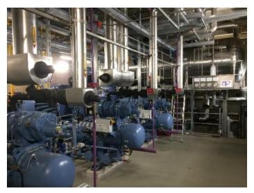
3 x SRM2016LS open-drive compressors packages with a displacement of 1270 m3/h are operating at up to 4200 rpm to ensure fast pulling down of the produce in the freezer.
