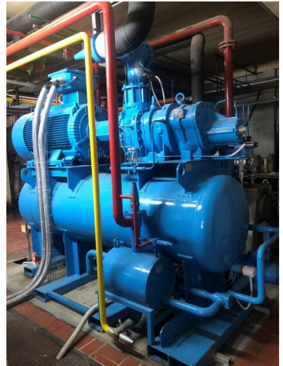
1 x SRMTec open-drive package with Qo: 974 kW capacity, horizontal oil separator and plate in shell oil cooler
