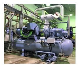
1 x SRMTec SNA26M-HAMA open-drive compressor-pack with Qo: 1500 kW capacity generates the ice for an ice bank to be ready for the quick pull-down of raw milk being delivered with trucks to a temperature of 6 °C to reduce germs growth.
