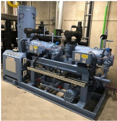
1 x SRMTec C2AA10L-VDHV semi-hermetic duo-compressor-pack with Qo: 320 kW capacity. Vertical oil separator, economizer and oil cooler
