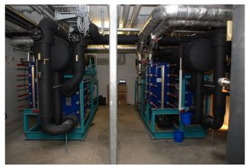
2 x SRS12L semi-hermetic compressors with a displacement of 287 m3/h each are operating on a common frame together with a plate heat exchanger as a chiller to deliver brine at exactly -6 C for stable process conditions.
