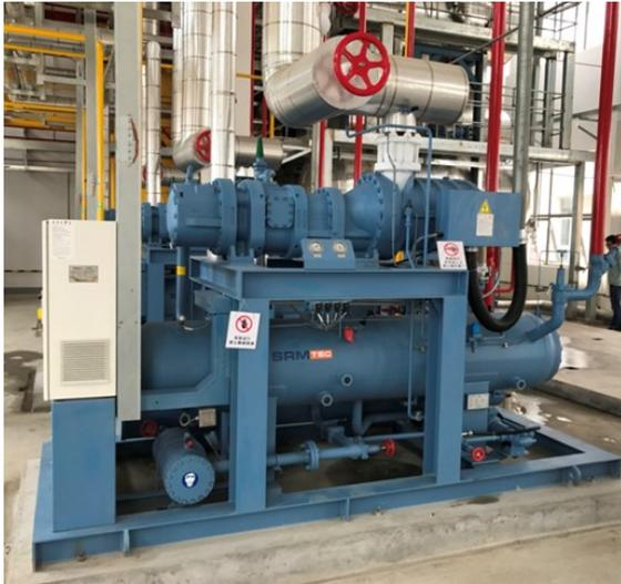
2 x SRMTec CAA1612LS-HALV semi-hermetic two-stage compressor packs with Qo: 550 kW capacity are operating via CO2/R744 as secondary coolant storage temperature zone -35° to -25 ° C. The fully welded plate-in-shell heat-exchangers of Vahterus are used for highest safety.
