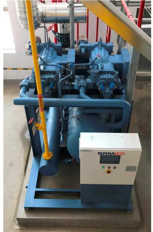
1 x SRMTec C2NA16L-HAHV semi-hermetic duo-compressor-pack with Qo: 695 kW capacity cools via propylene glycol as coolant the storage temperature zone 0 bis 12 ° C.
