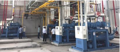
The first semi-hermetic installation was the BRAUNLAGE ice rink in Germany in July 2017 where the semi-hermetic screw compressor fitted perfectly to this application:
