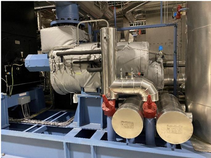
High efficient Plate Heat Exchangers, Motors, Insulation, optimized Piping reduce refrigerant charge and increase system efficiency whereas dual oil filters, oil temperature regulation valves and other control devices assure smooth operating and process security.
