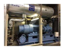
The heat pump is controlled by Siemens S7 PLC and regulates the capacity in co-relation between VSD and the mechanical slider according to the demand of heating energy. With its high COP of 3.8 in combination with the
