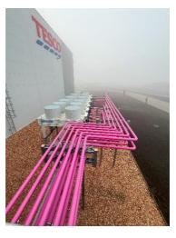
The high temperature packages provide with 3 compressors up to 550kW cooling each at -6°C and a condensing temperature of +50°C.
